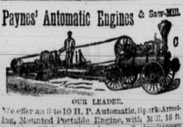
carriage, 32 ft. track and ways, 2 simultaneous lever set head-blocks, 24-inch arbor, 3 changes feed: sawyer controls feed-lever and head-blocks from one position. 50 inch solid saw, 50 ft. 8 inch 4-bly belting, feed-belts, cant-books, sware, tightener, etc. Hig complete for operation, \$1100 on cars, Engles on skids, \$100 leas. English shifted and the saw two
